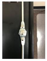
With the rods located inside of the nylon guides top & bottom, position the cam and locking rods so they resemble those in the photo, in a straight line. At this point make sure the the rods are protruding through the top and bottom of the door.
